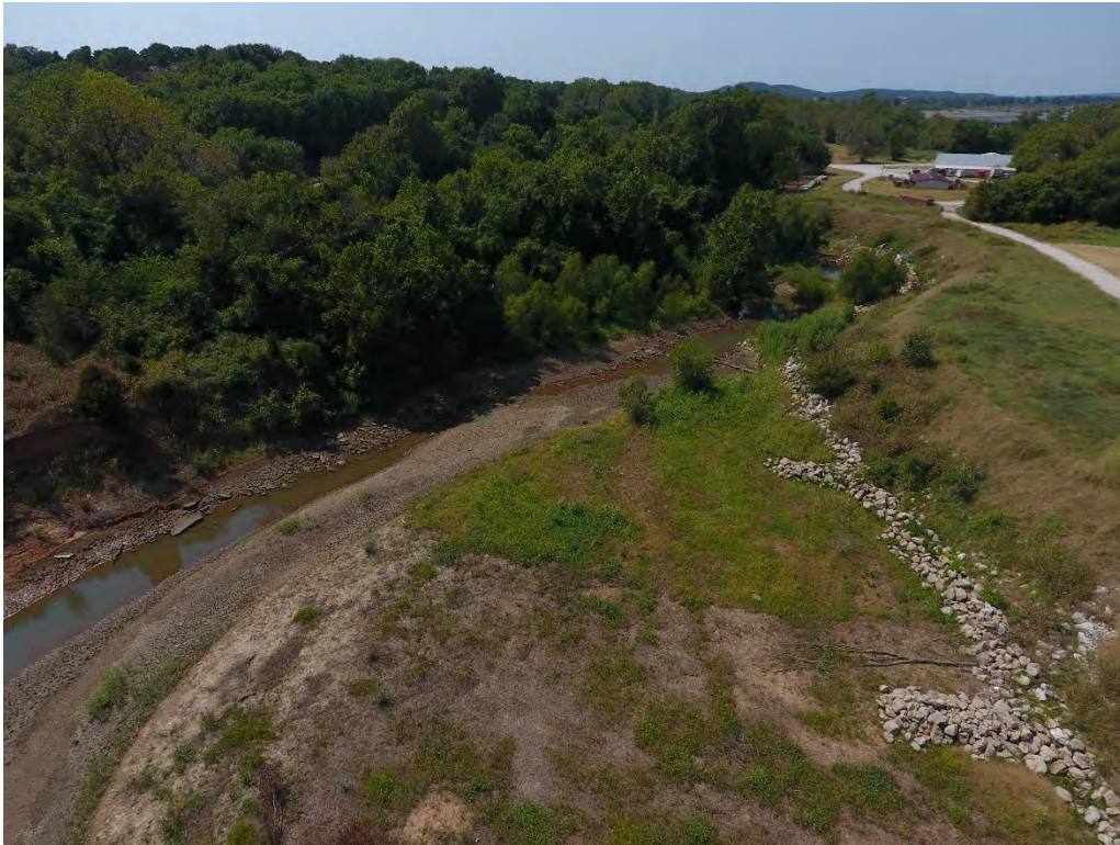
Figure 13. Drone Photograph--Prattville Creek Looking Upstream at Sand Springs FFA Farm
